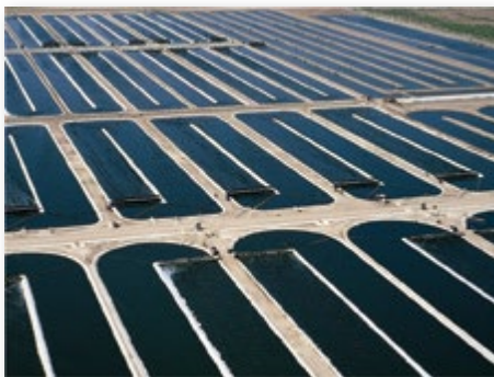
▲ Figure 3.1: Large-scale open ponds at Earthrise farms, California, US
