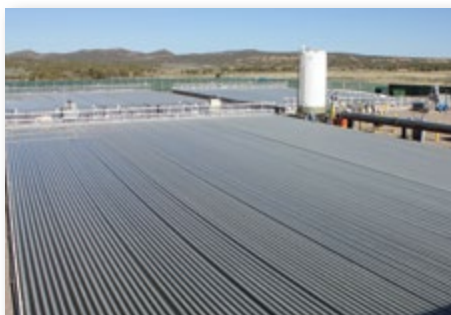
▲ Figure 7.5: Demonstration plant of Solix in southwestern Colorado, USA
